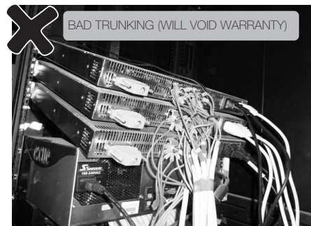
FIG.9: Bad vs. Good trunking. It is recommended to follow the example on the right.
