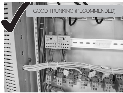
FIG.9: Bad vs. Good trunking. It is recommended to follow the example on the right.
